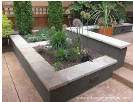
CONCRETE PLANTER - SEAT HEIGHT WITH PRECAST STONE CAP
