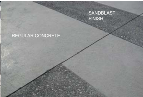
CONCRETE BANDING AND PLANTER - HEAVY SANDBLAST FINISH TO PROVIDE TEXTURE
