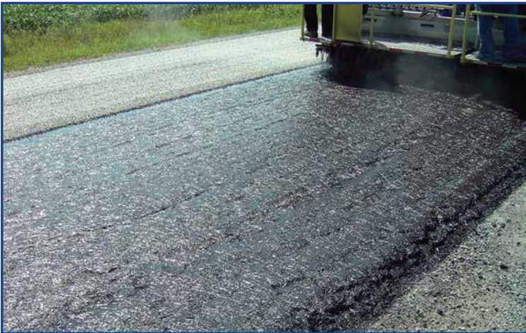
Placement of FiberMat™ membrane.
