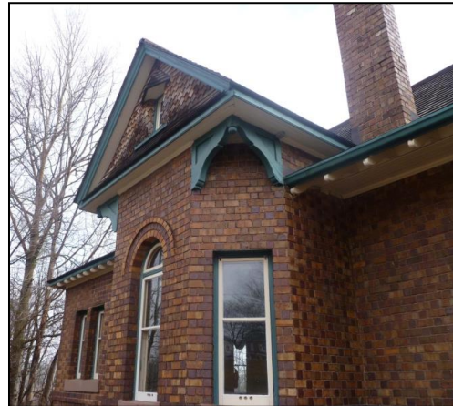
West facing gable with corner brackets, showing curved lintel and semi-circular light above west-facing window; shows position of chimney on roof.
