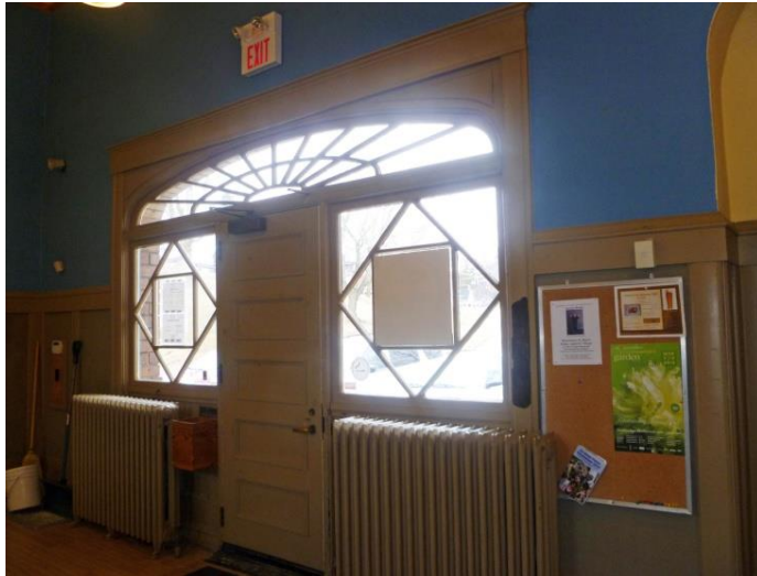
Interior view of main west-facing entrance showing elliptical fan light over five-panel door flanked by windows and panels (behind radiators); also shows wide casing, wainscoting and ledge.
