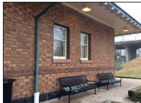
Two views of overhang on west side, soffit and curved brackets; Good view of brick pattern – Flemish bond.
